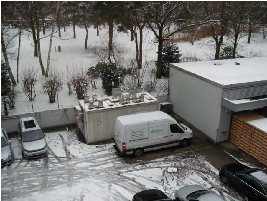
Figure 32: Field test site Cologne, summer & winter
