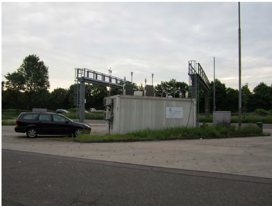
Figure 34: Field test site Bornheim, summer
